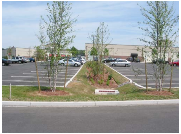
Figure 6. Bioretention practices used to accept and treat stormwater from parking areas in Portland, Oregon (left) and Evergreen Walk Mall in Manchester, CT (Right).
