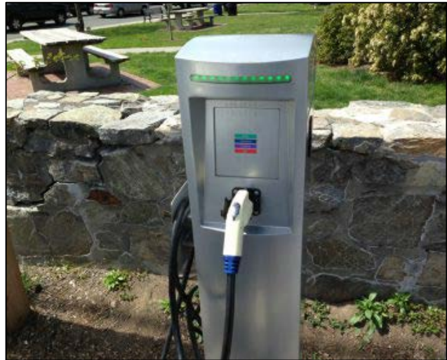
Figure 5 Fairfield has four Level 2 electric vehicle charging stations in Town. Visible charging infrastructure is important to the mind-set of the potential EV consumer.
